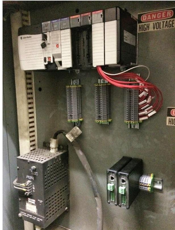
Thanks to the gateway, the ControlLogix is able to control the SY/MAX I/O. In the long-term, the company is planning to replace the remote racks, but this phased modernization has enabled them to do the work on a timetable that makes sense for American Castings and its business goals.
